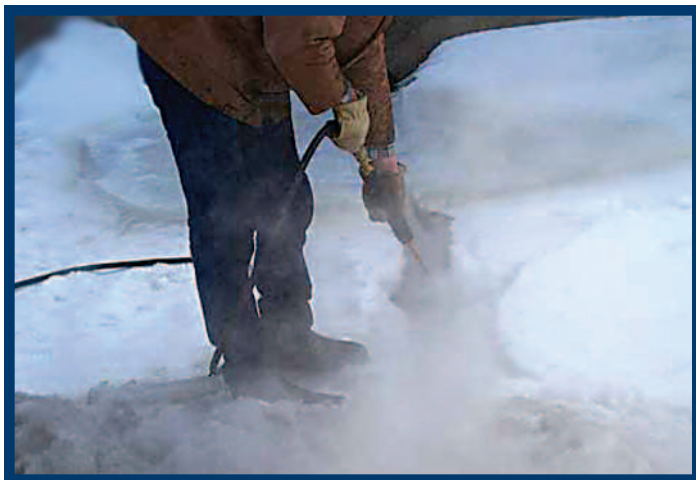
Easily melting ice dam for drainage
